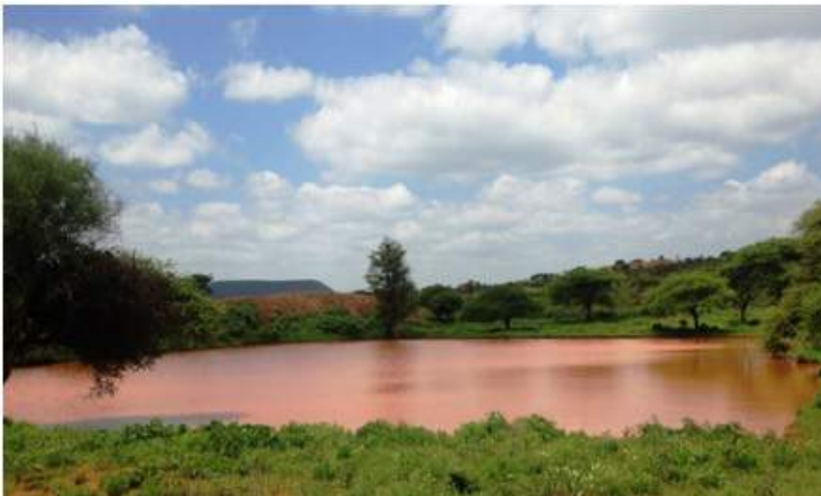
Figure 5: One of the four new ponds constructed by ACORD in its livelihood project (Dida Jarsa kebele, Dire district)
